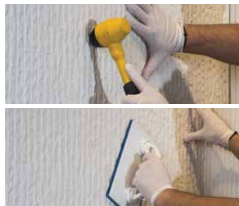
5. The panel is mounted on the wall, and the assembly process is completed with the help of a plastic hammer and sponge trowel to ensure it is firmly fixed.
